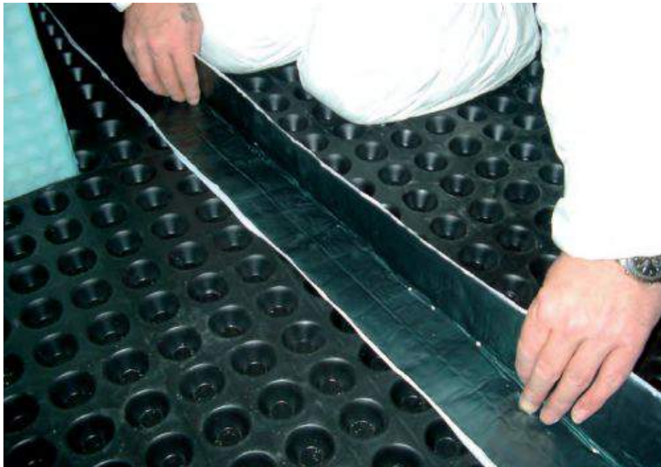
FORMING 90° ANGLE CREASE IN CORNER STRIP
