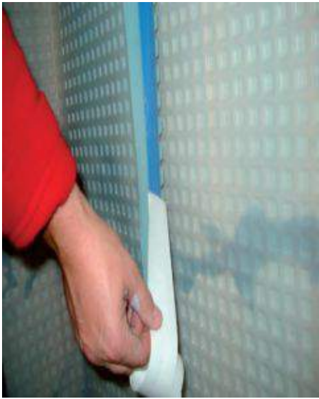
P20 FLOOR MEMBRANE CUT AROUND PERIMETER WALLS
